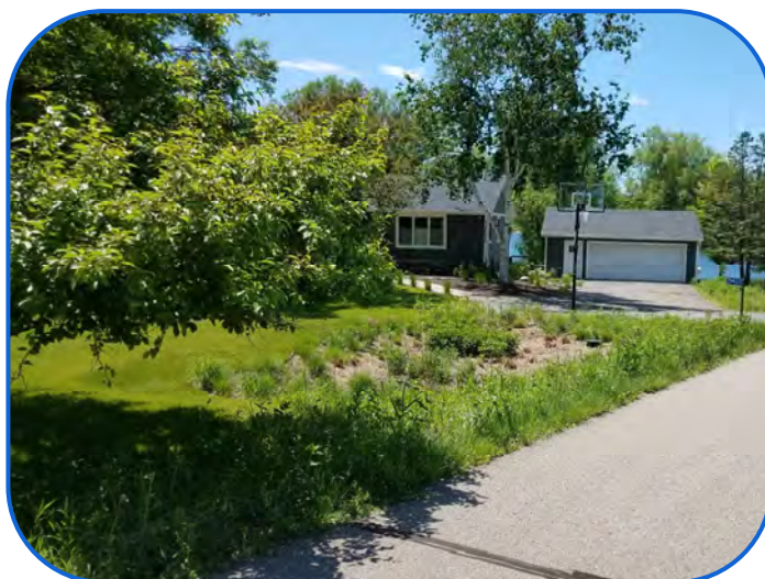
Infiltration Area After Project Completion
