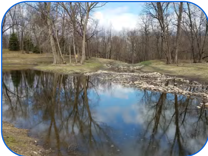
Gully Area After Construction
