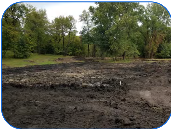
Wetland Area During Construction
